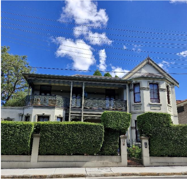
Wyandra, 12 Elizabeth Street, Ashfield
